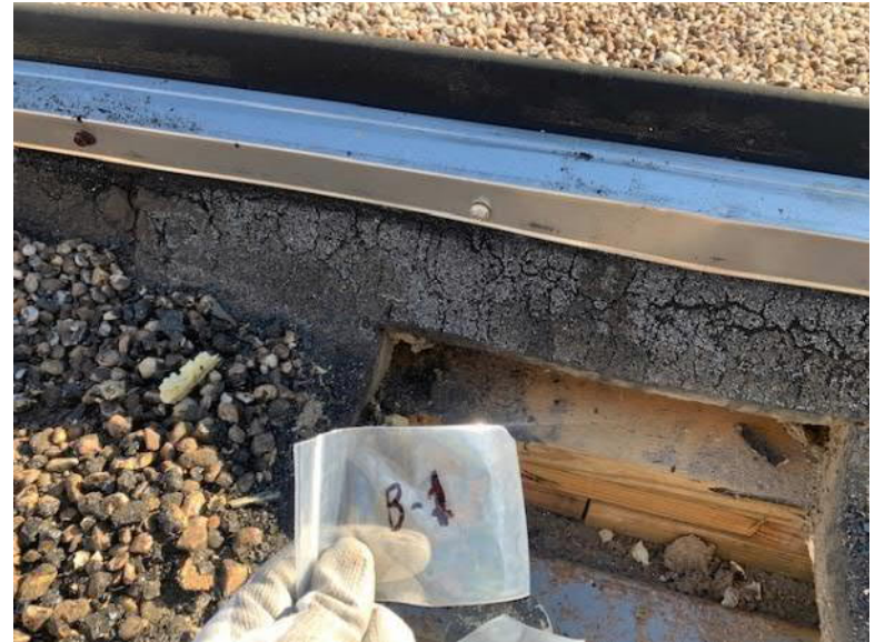
Photo 2: View of base flashing
