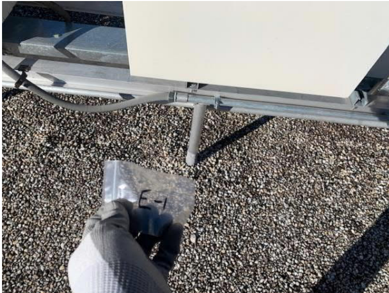
Photo 5: View of gray penetration flashing elevated HVAC racks.
