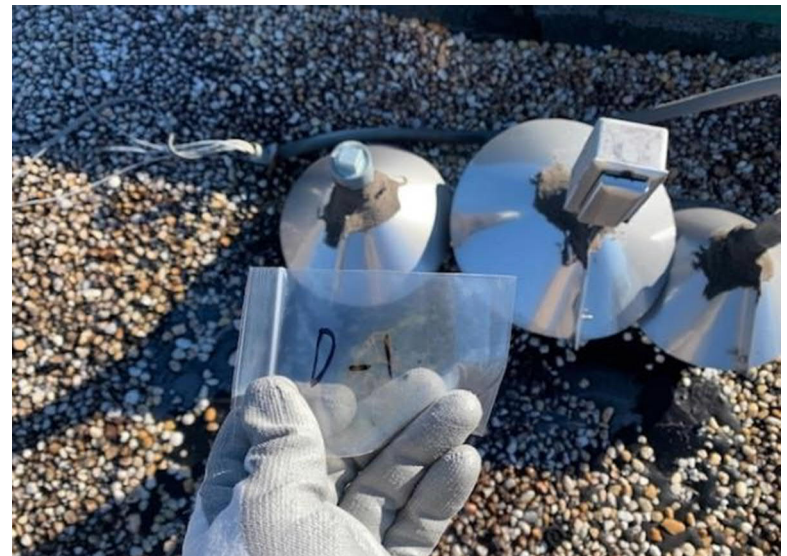
Photo 4: View of black penetration flashing.
