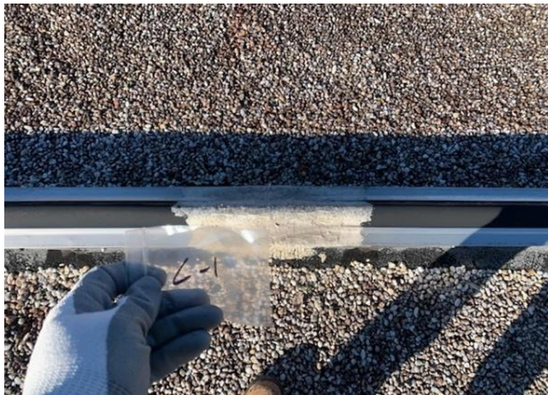
Photo 3: View of white sealant on main roof expansion.
