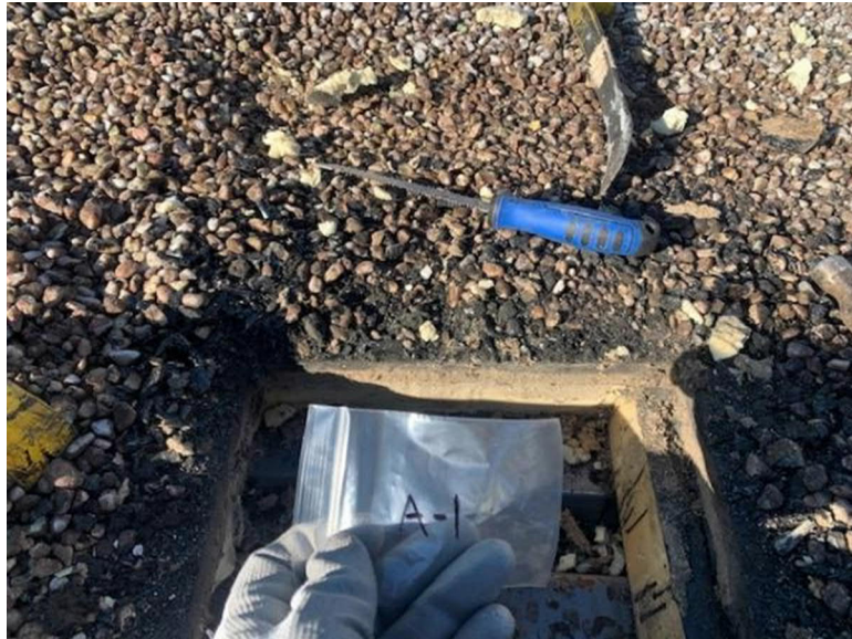
Photo 1: View of built-up roofing field.
