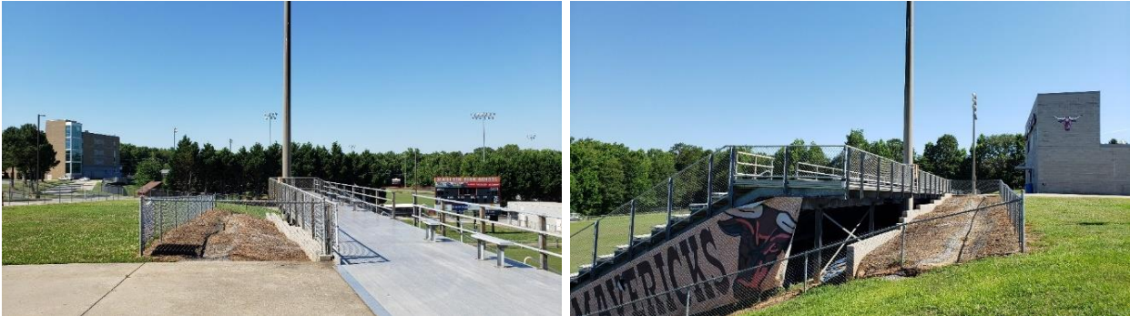
Images Below | Shown are the current bleachers on both the home and away sides. Both sides will be expanded to accommodate more spectators. The home side bleachers will require retaining wall expansions and enhancements to support the additional seating on either side. Additionally, improvements will be made to address erosion issues under the existing stadium seating, ensuring long-term stability and safety. These upgrades will significantly increase capacity and improve the overall spectator experience.
