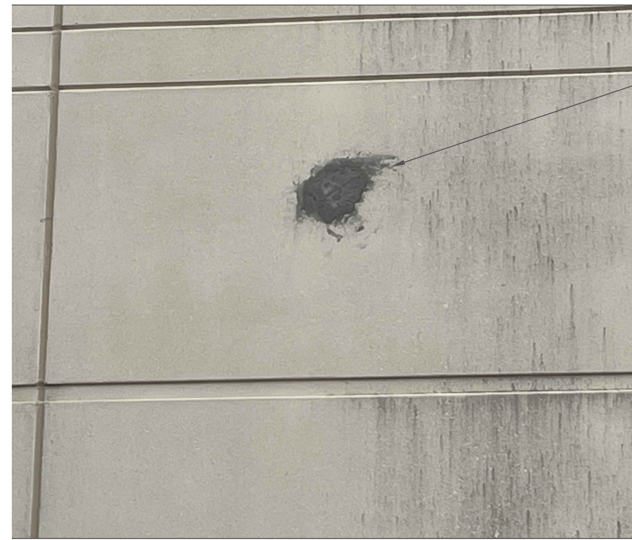
1 CONCRETE PATCH REPAIR - PRECAST SECTION C-7 SCALE: NONE
