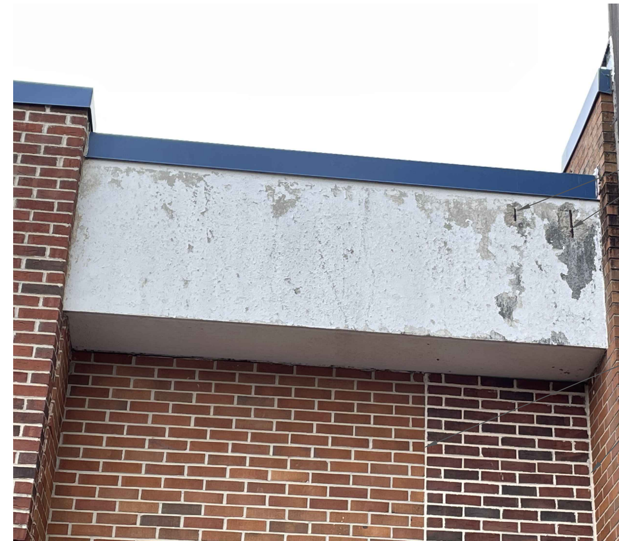
2 CONCRETE REPAIR - PRECAST SECTION C-7 SCALE: NONE
