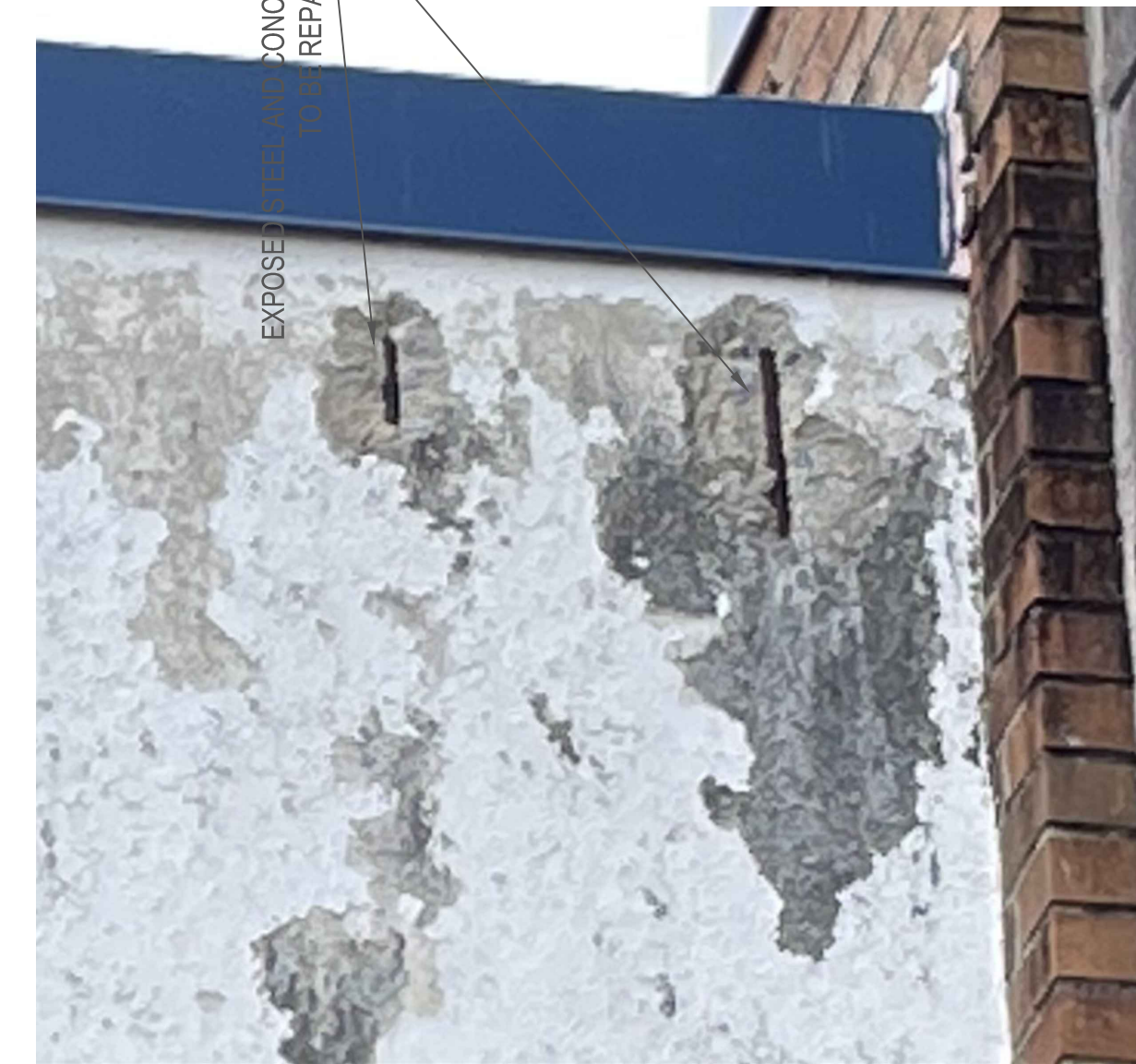
3 ENLARGED CONCRETE REPAIR C-7 SCALE: NONE
