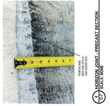
2 CONCRETE REPAIR - PRECAST SECTION C-7 SCALE: NONE
